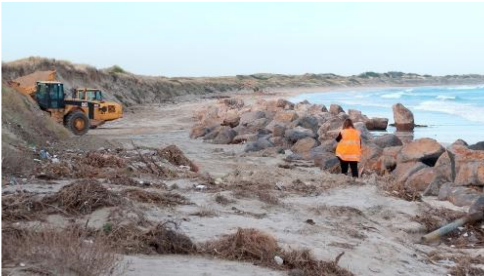
Figure 12- Council landfill site looking to north east exposed due to dune erosion after 2015 storm event with WEDS in foreground
