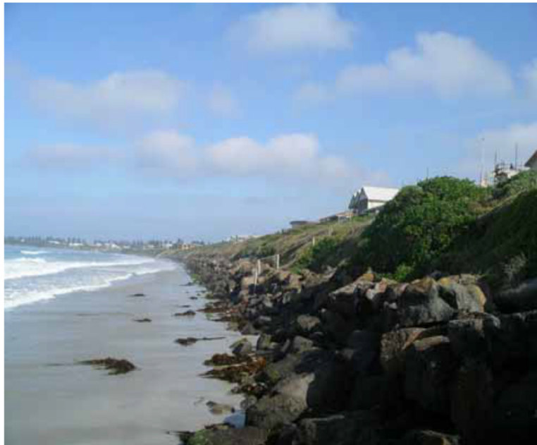
Figure 9- Photo of rock revetment looking to the south west. This section of the revetment was repaired and upgraded in 2012 BMT WBM (2007)
