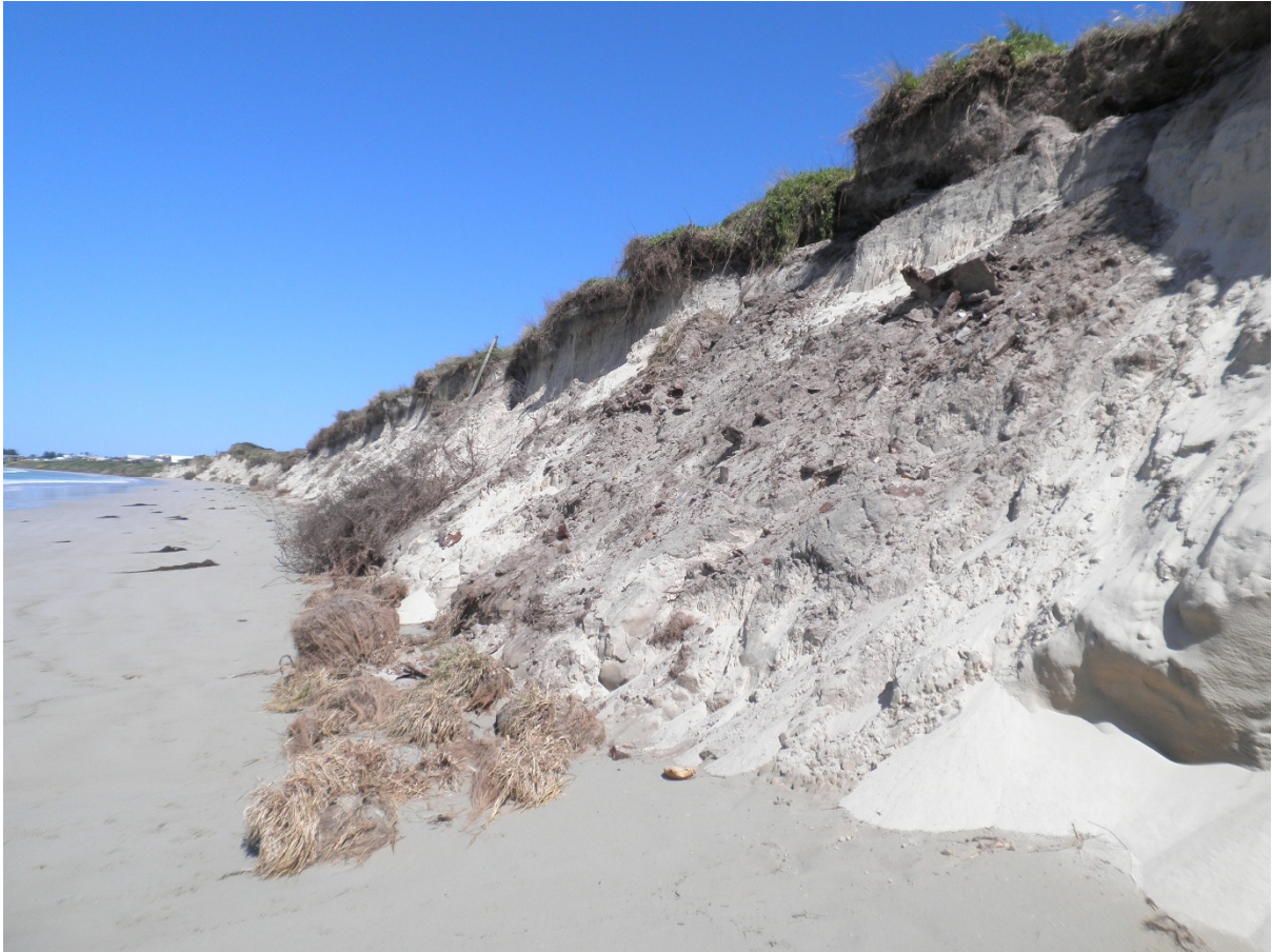
Figure 11- View of active dune erosion to the south west of the DELWP landfill site in November 2011 after storm damage
